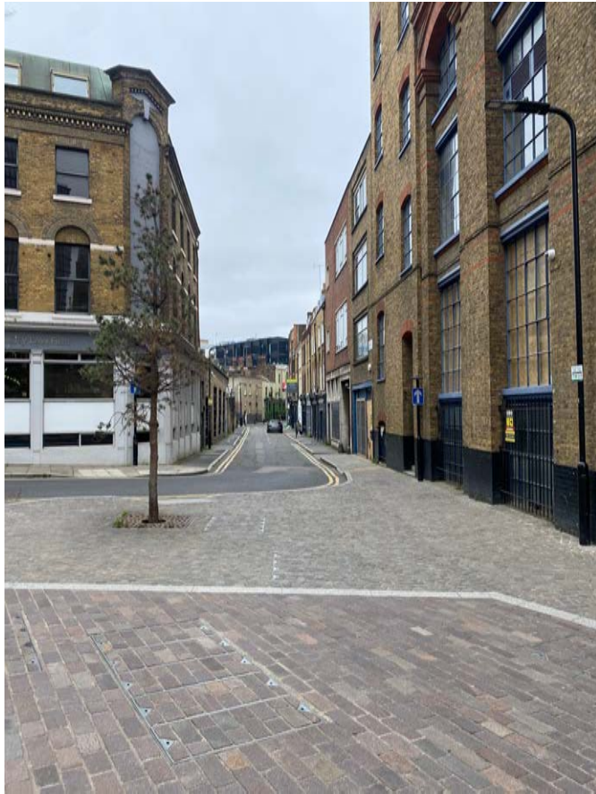
Clifton Street towards Holywell Row
